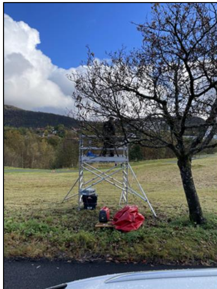
Figure 89. Camera operator on scaffolding and the camera rack on the floor (camera 5).
