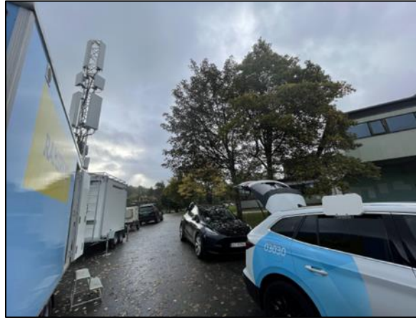
Figure 86. Cell with 2.3 GHz and 3.6 GHz antennas placed.
