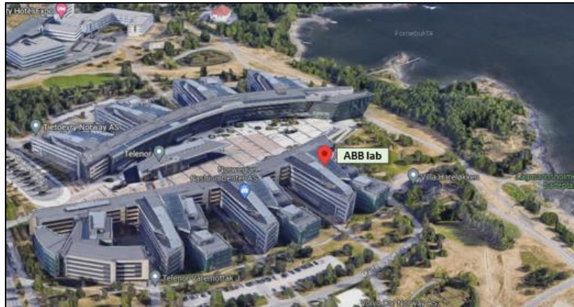
Figure 39. ABB premises location in Fornebu, Norway.
