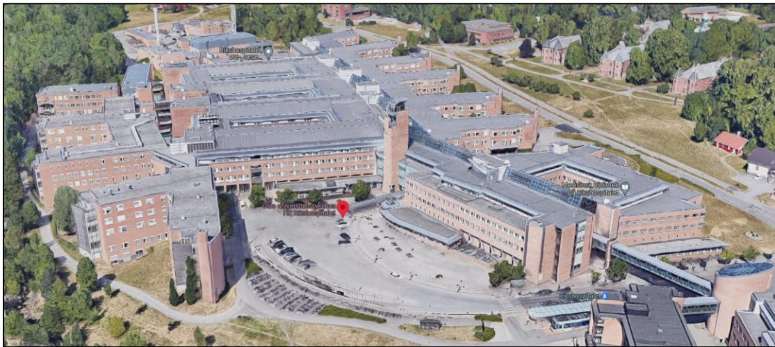
Figure 23. Oslo University Hospital
