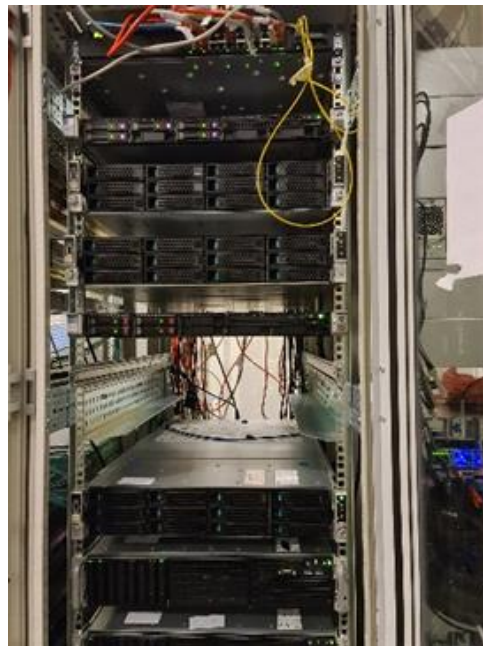
Figure 7: Central computing server rack in Fornebu experimental network.
